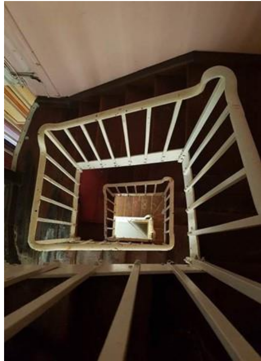
Plate 195: View down winding staircase
