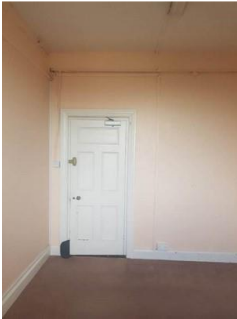
Plate 147: A typical dormitory in main corridor with modern door and architrave
