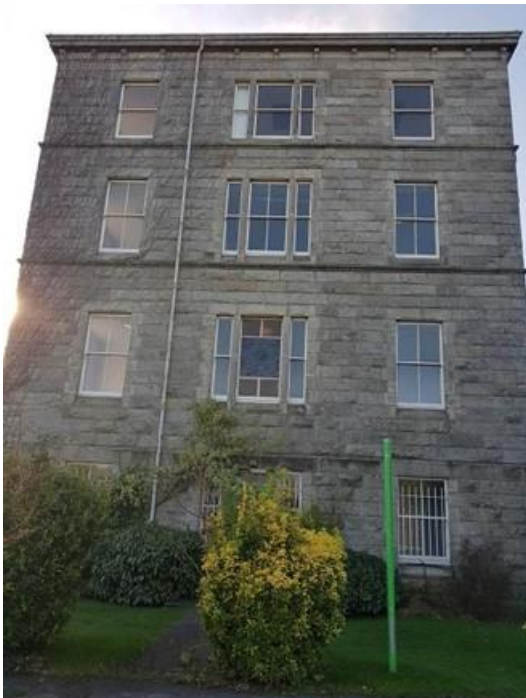
Plate 25: North east gable elevation of Tabor House
