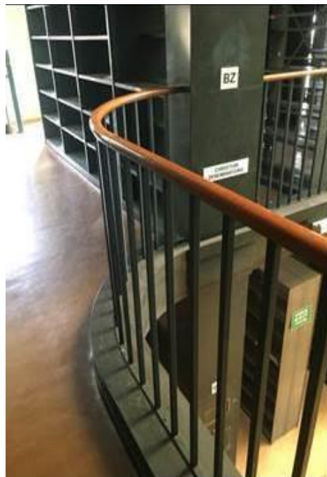
Plate 270: Detail of curved handrail at end floor mezzanine level
