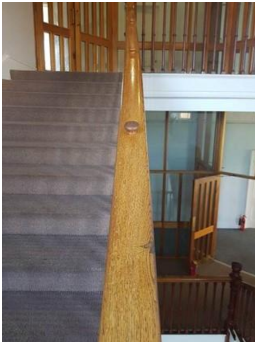
Plate 208: Detail of oak handrail
