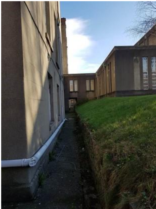
Plate 14: Trench at base of lower ground of rear extension
