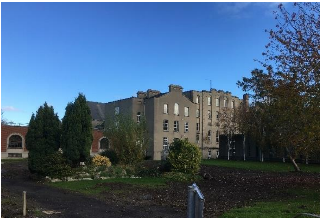
Plate 17: Southwest view of the rear extension
