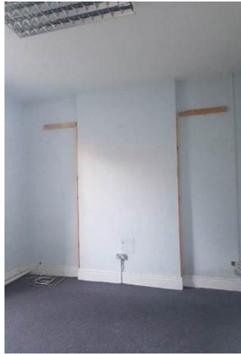
Plate 175: Lecture room, without fireplace
