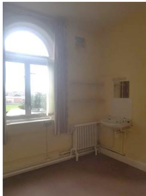
Plate 146: A typical dormitory with replacement arched window
