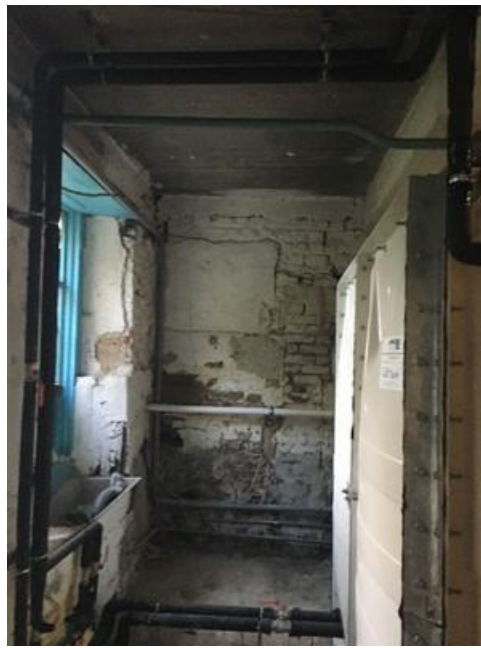
Plate 105: View east in same room
