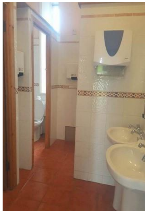
Plate 138: Toilet block within 1 st floor level
