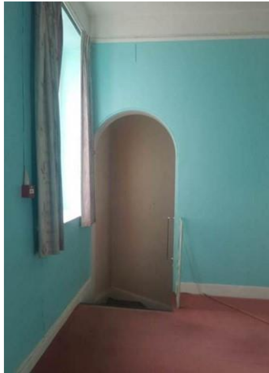
Plate 107: Archway leading to stairs to entrance level
