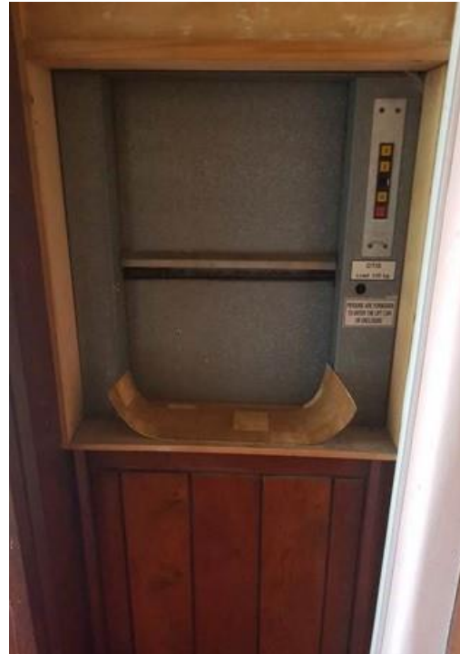
Plate 187: Dumb waiter from kitchen to dining area
