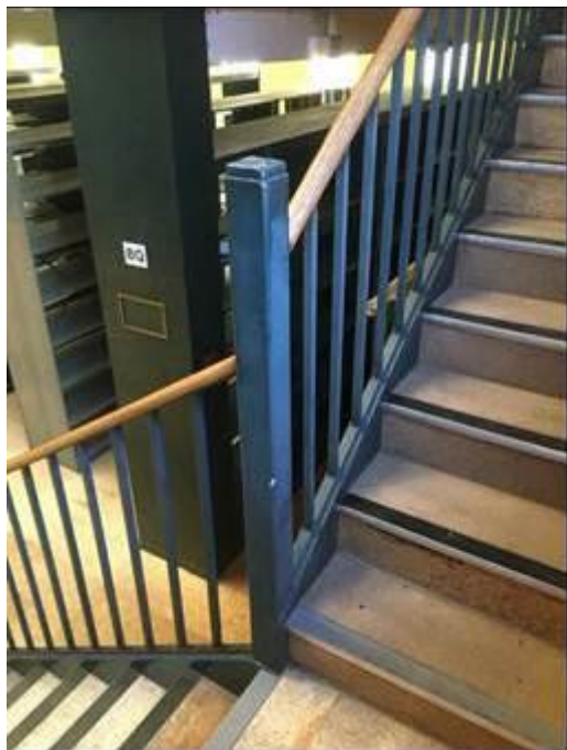
Plate 269: Detail of stair steel banister and oak handrail
