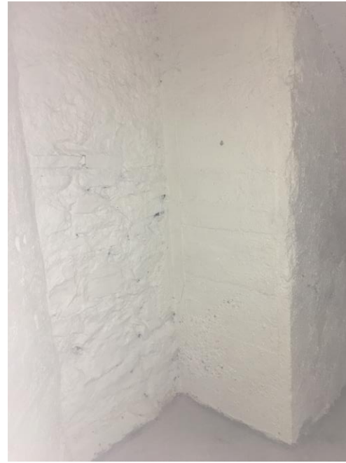
Plate 101: Historic masonry pier
