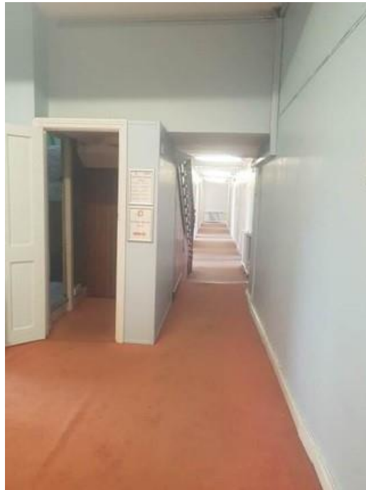
Plate 117: Central hall at 2 nd floor level linking to rear extension block. Note water tank room to lhs of image which extends up into roof void
