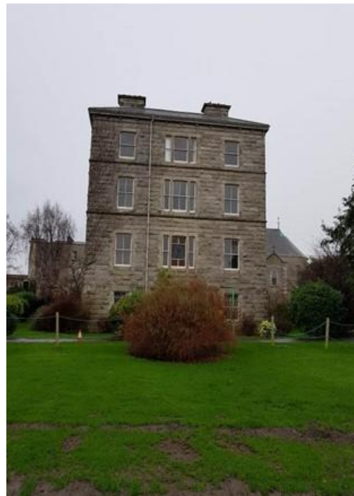
Plate 22 : North-east gable of Tabor House in context
