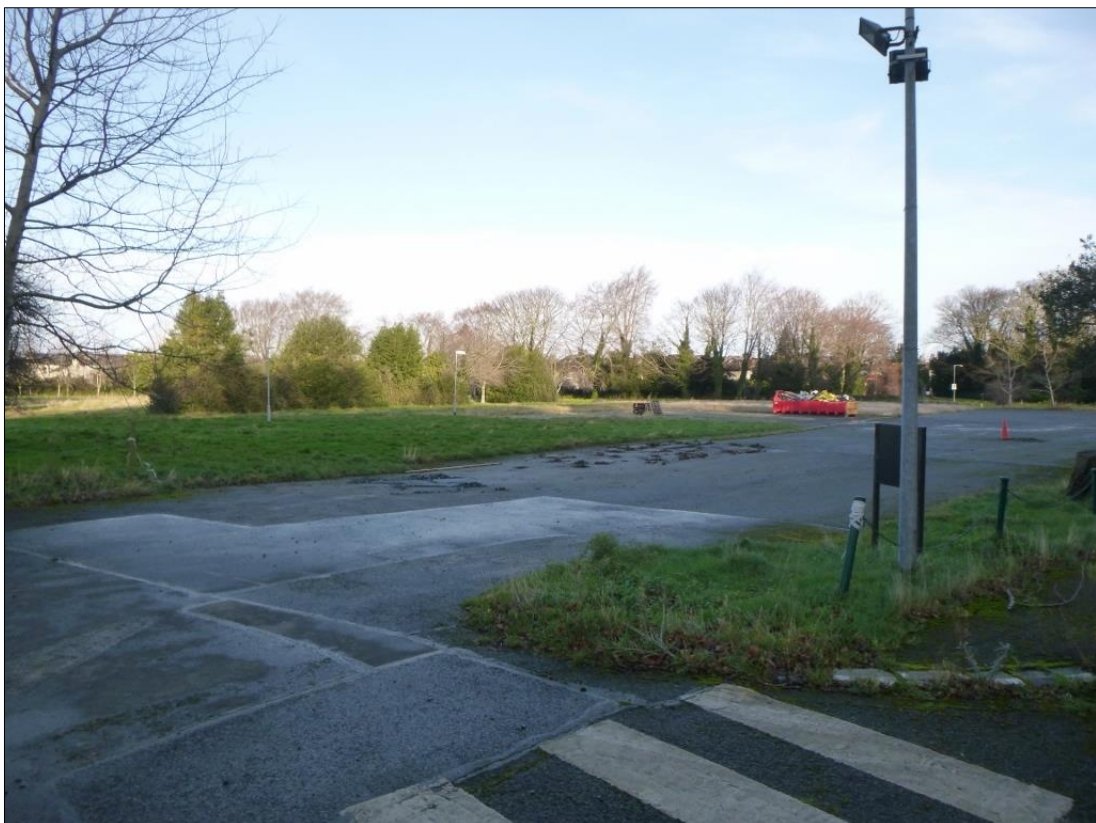
OVERALL VIEW OF PROPERTY – NORTH CENTRAL SECTOR, LOOKING NORTH WEST
