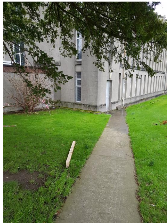
Plate 59: East elevation, gable to south
