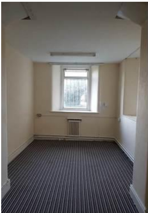
Plate 234: Typical basement room
