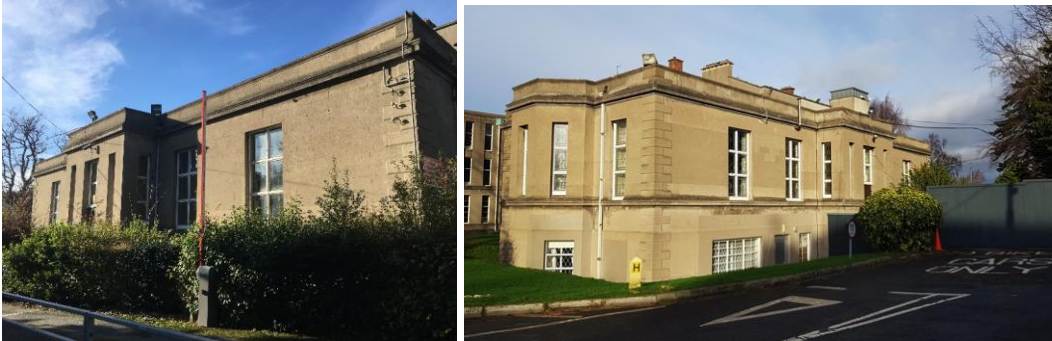
Fig.39 Views of east elevation
