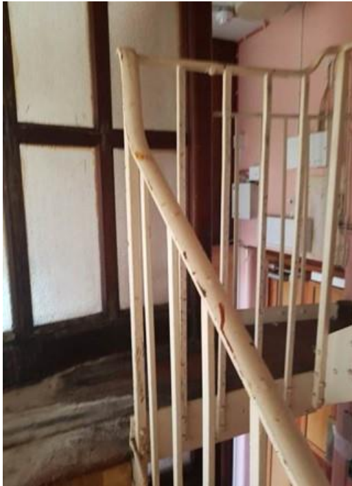
Plate 194: Service staircase of wood and iron
