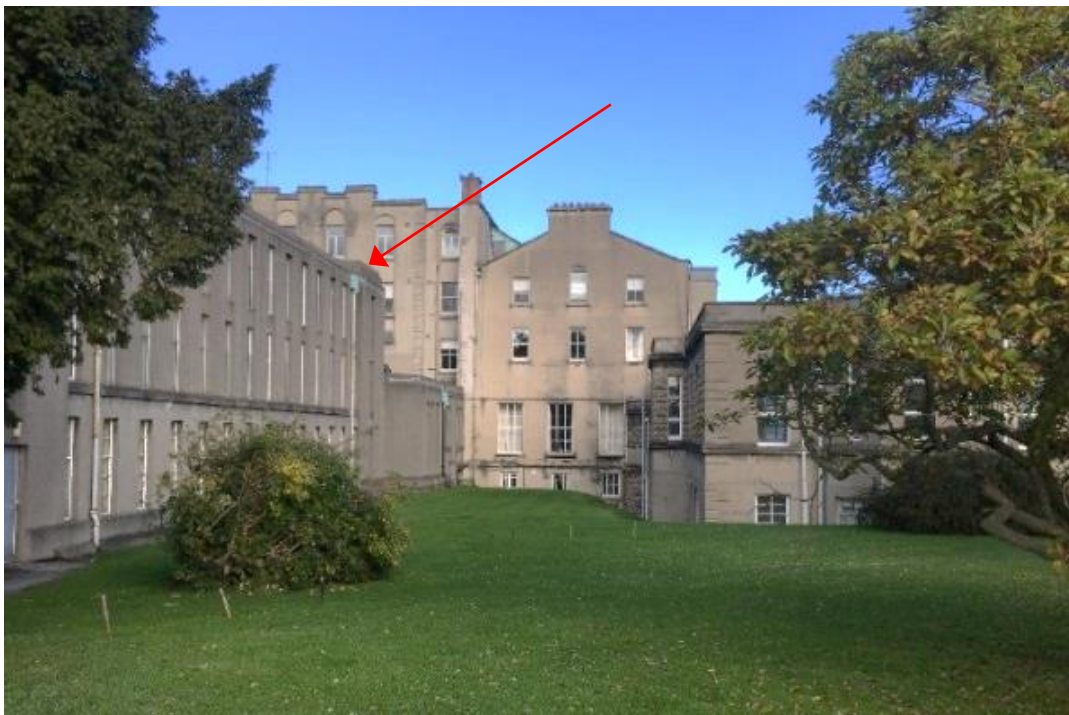
Plate 53: Southern elevation of Milltown house with Archive wing in context
