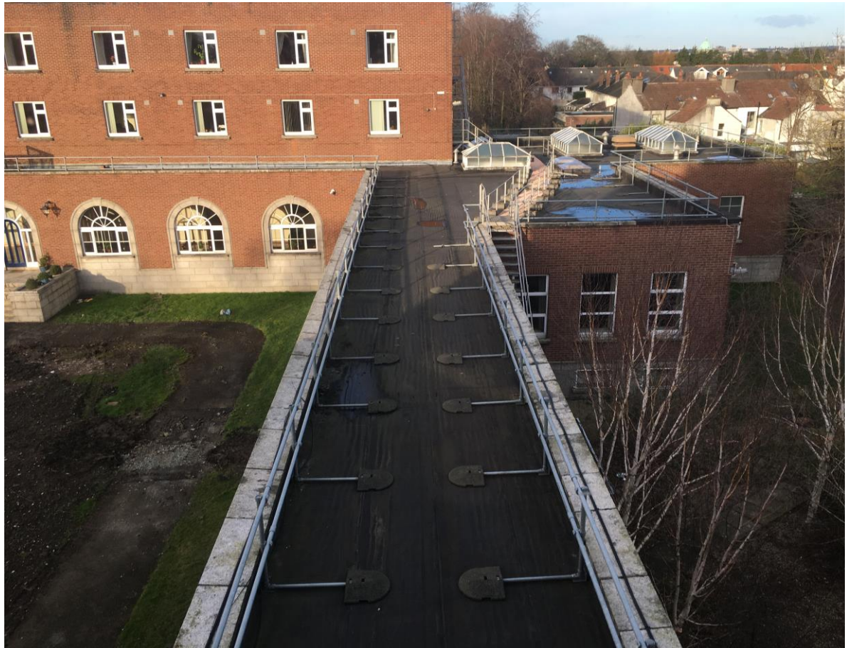
Plate 66: The flat roof arrangement over the red-brick link building, as viewed from stairwell of Building B
