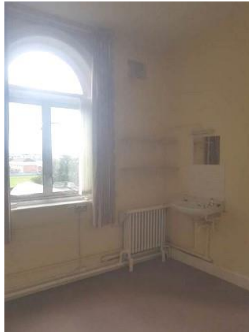
Plate 163: Apsed window in bedroom to southwest
