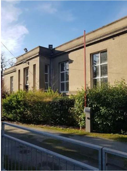
Plate 41: View of Finlay wing, south west from the main entrance
