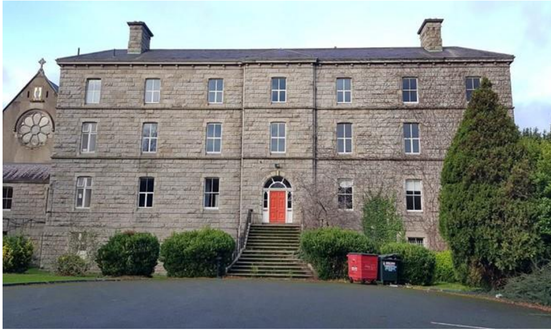
Plate 18: Front elevation of Tabor House with chapel and stained glass window in view
