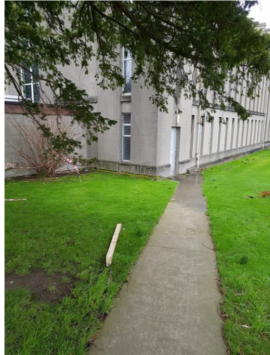
Plate 50: East elevation, gable to south
