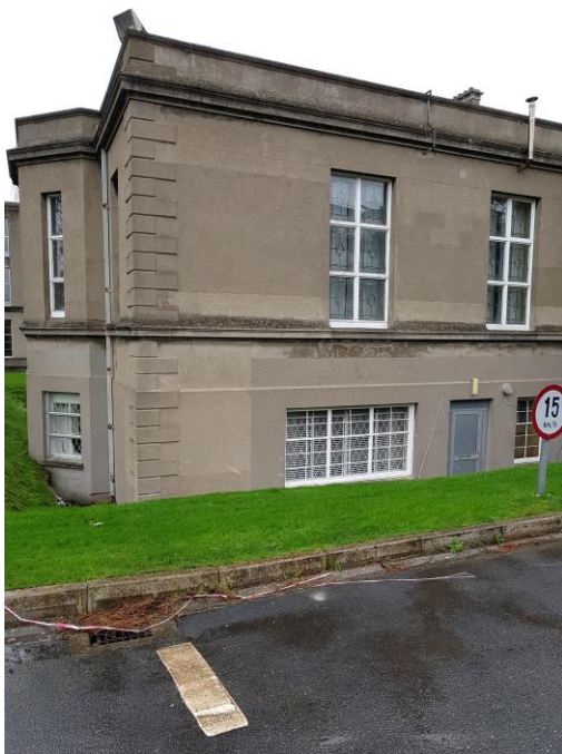
Plate 43: Eastern elevation of Finlay wing
