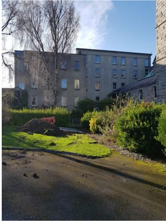
Plate 9: North east gable of rear extension block in context
