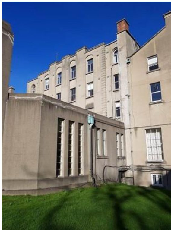
Plate 7: Southern elevation showing connection to Rear Extension and Archive
