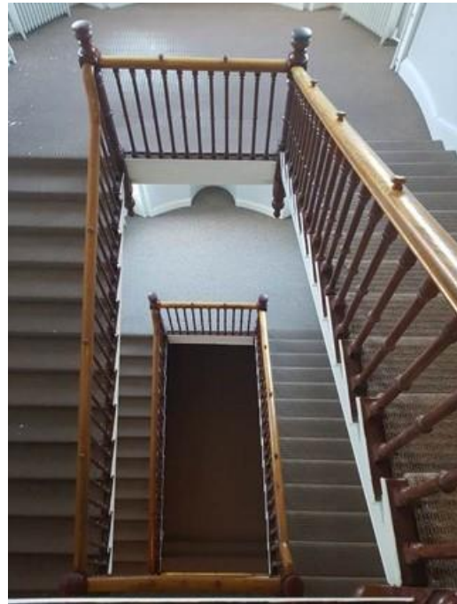
Plate 207: View down central stair
