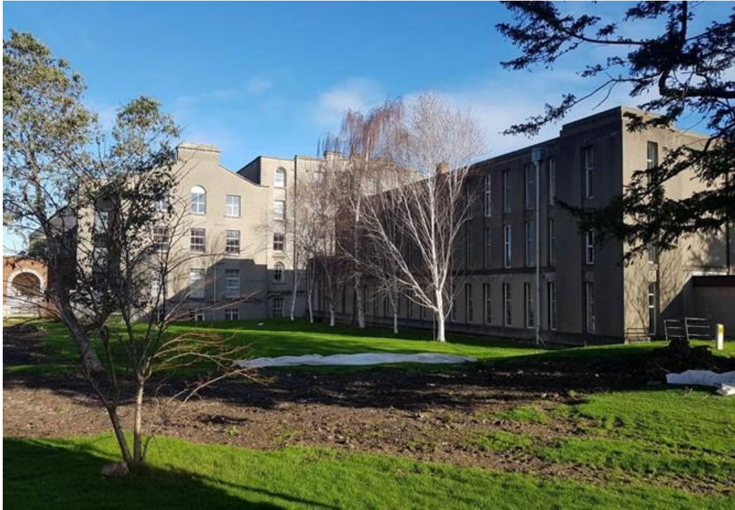
Plate 60: NW elevation of archive with 19 th c. rear extension in background
