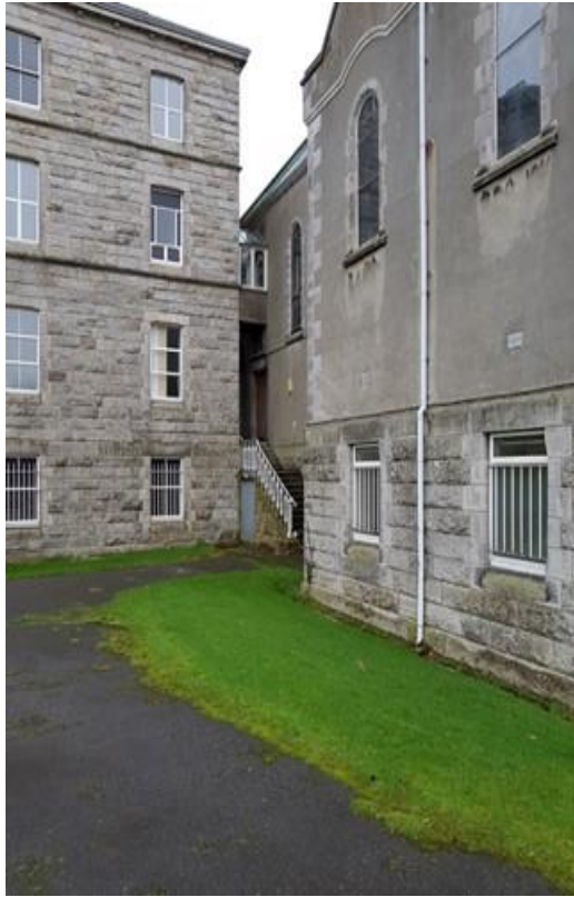
Plate 27: Connection of Tabor House to the later Chapel: comprising a set of stone steps to first floor level, and a glazed link at second floor to the mezzanine at the rear of the Chapel
