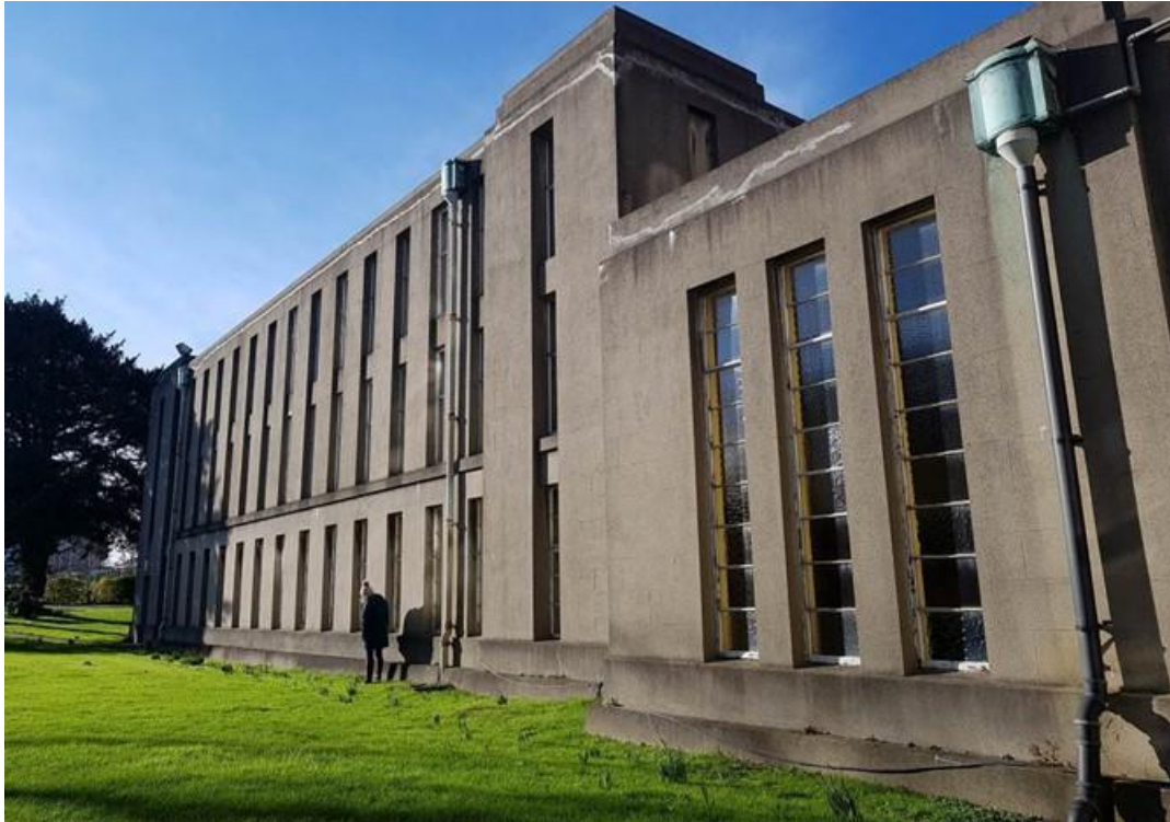
Plate 52: SE elevation of Archive wing. Original 1930's window frames. Copper hoppers to rainwater goods, Art deco detailing of parapet walls
