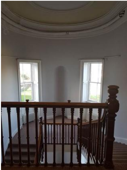
Plate 206: Return at top of central stairs
