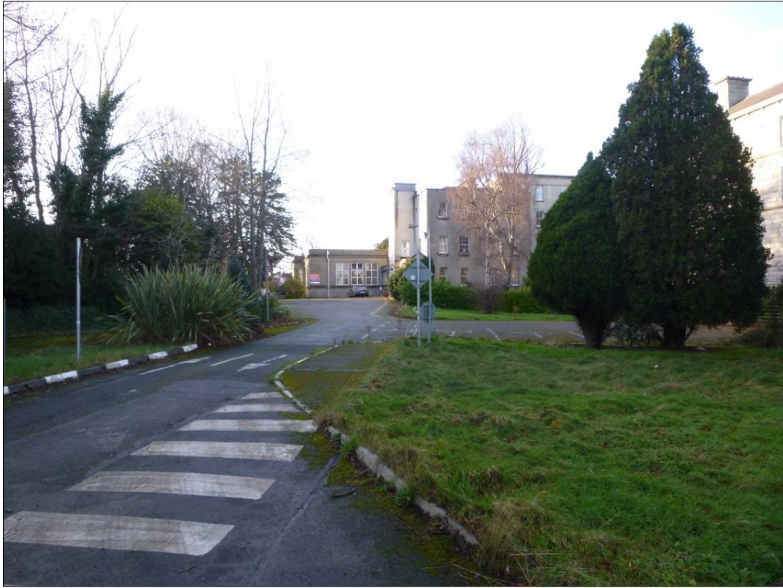
OVERALL VIEW OF PROPERTY – SOUTH EASTERN SECTOR, LOOKING SOUTH
