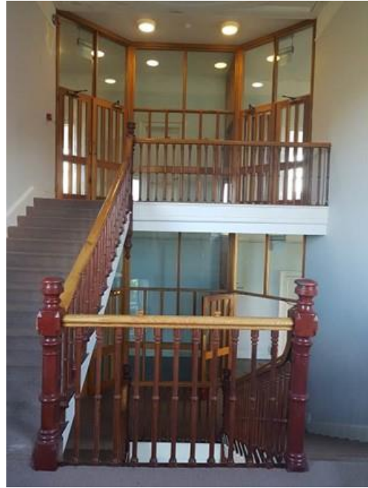
Plate 211: View from second floor landing to third floor with glass door screen to corridor
