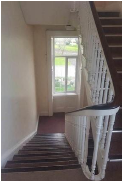
Plate 168: Painted stair to rear of block
