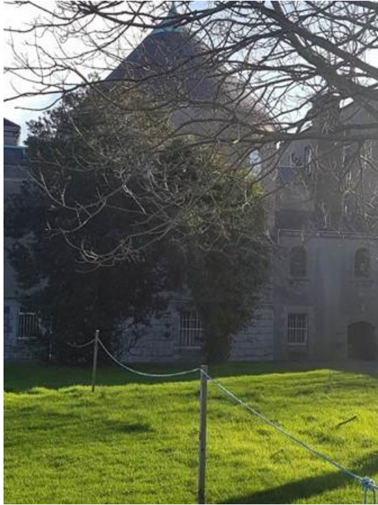
Plate 32: Rear of Chapel and copper turret
