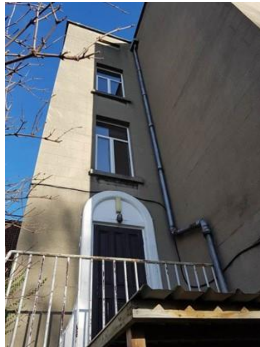
Plate 15: Panelled door to rear entrance of rear extension, late 19 th century
