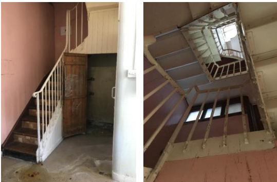
Fig.65 Secondary steel stair of interest
