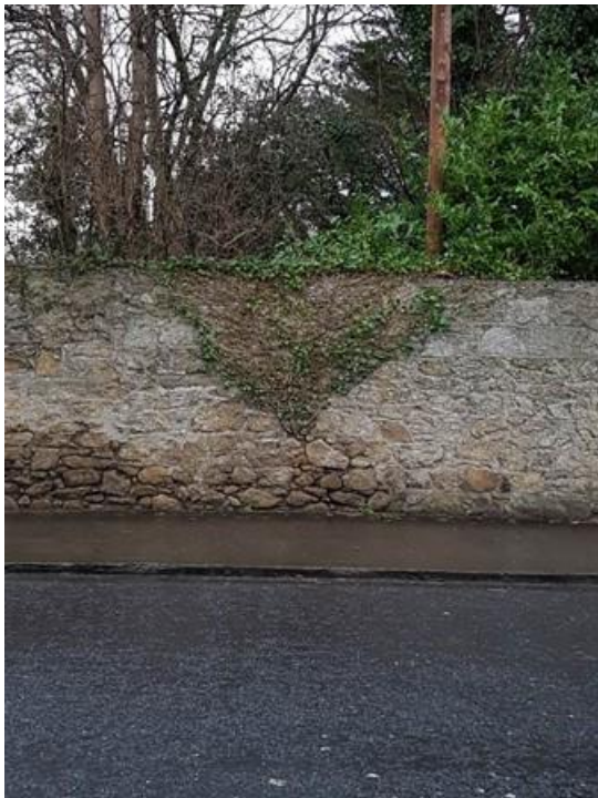
Plate 71: Section of rubble boundary wall on Milltown Road
