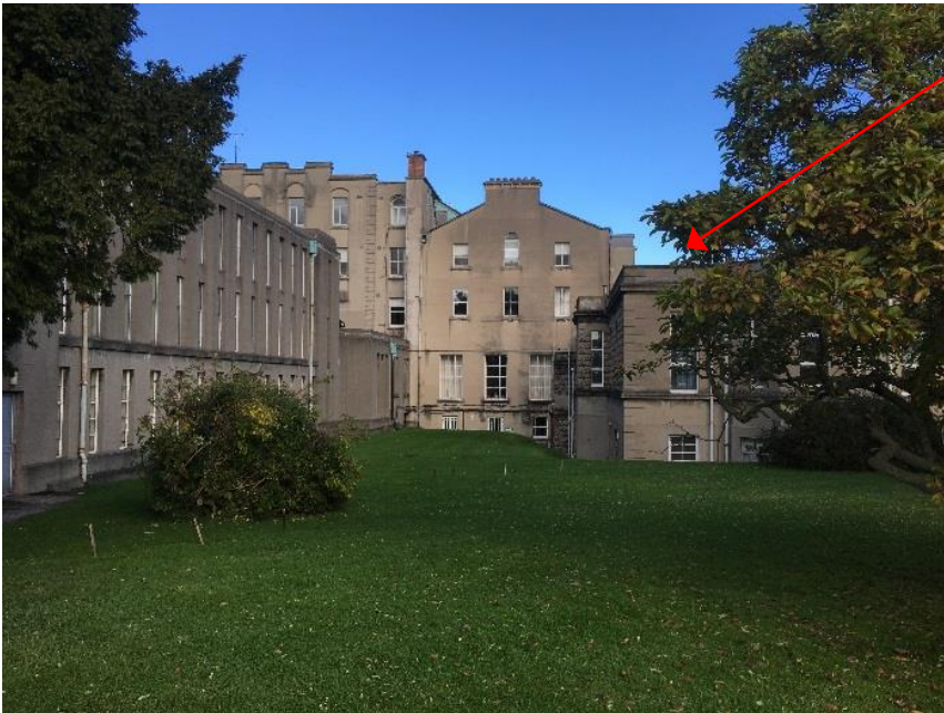
Fig.40 View of south elevation (behind tree) as demarked by arrow
