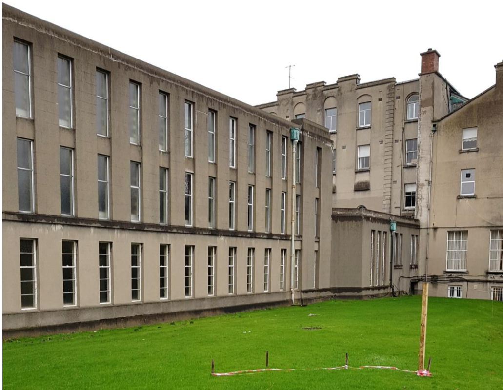
Plate 54: SE elevation of Archive wing where it joins the Rear Extension of Milltown Park House. This is the only point of entry which is internally via Milltown Park House and involves a series of level changes
