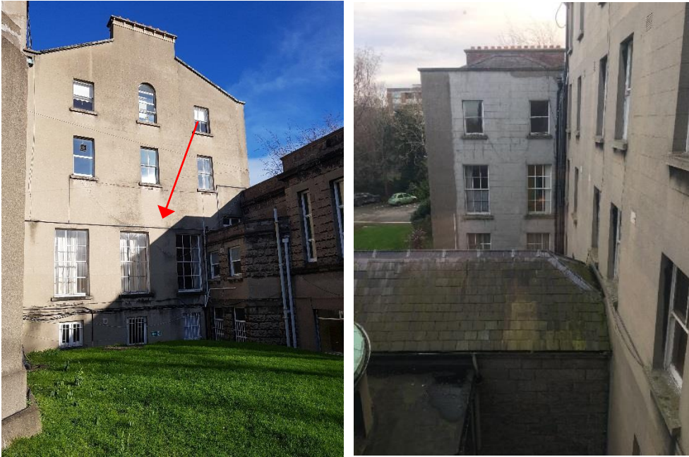
Fig.21 Southern elevation, comprising an extension, with its expressed gable in context with the Finlay Wing and Archive (corner visible). Lower windows are early in origin, with the 6/6 windows attached to a former orangerie, which was vertically extended in the 20 th century.
