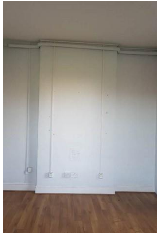
Plate 179: Chimney breast without fireplace
