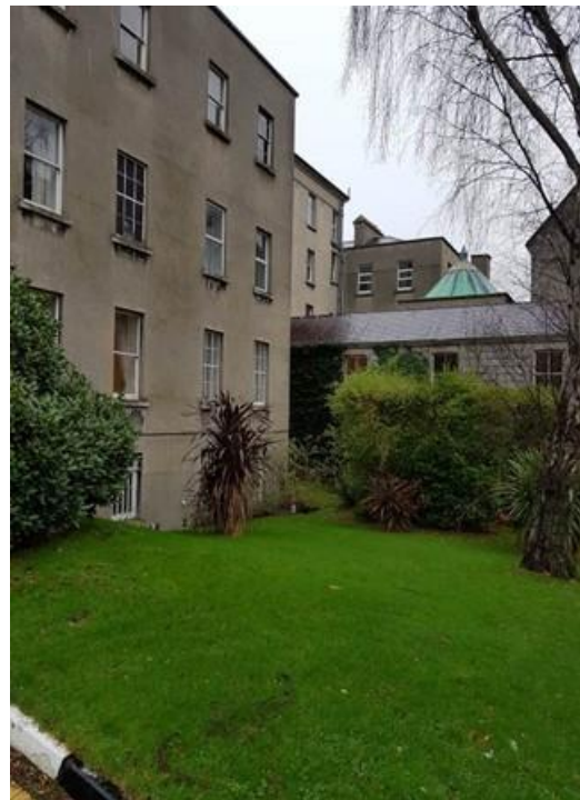
Plate 31: Link building connection to rear extension to Milltown house with small turret of Sacred Heart Chapel in view and larger domestic Chapel just out of view
