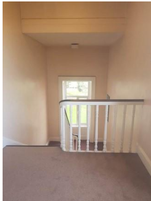
Plate 169: Second floor landing
