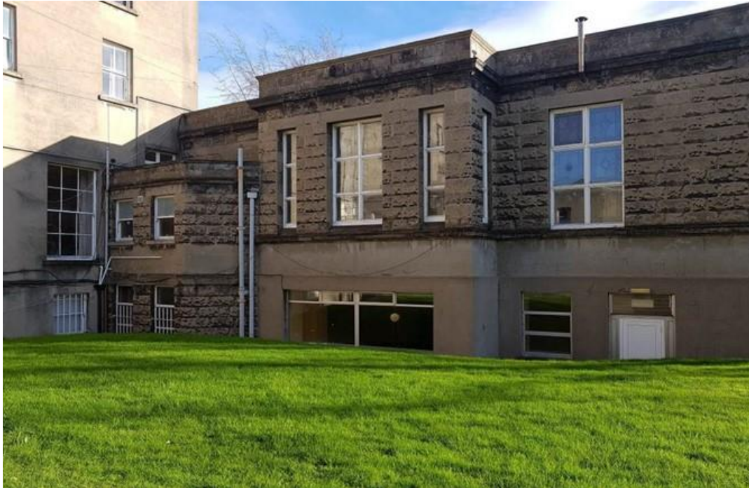
Plate 45: View of NW elevation of Finlay wing and awkward connection to Milltown House. Note stained window panes dating from post 1949 reconstruction
