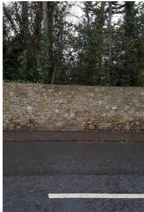
Plate 72: View of rubble wall and trees visible from Milltown Road
