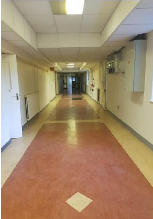
Plate 133: Same corridor, viewing from east to west
