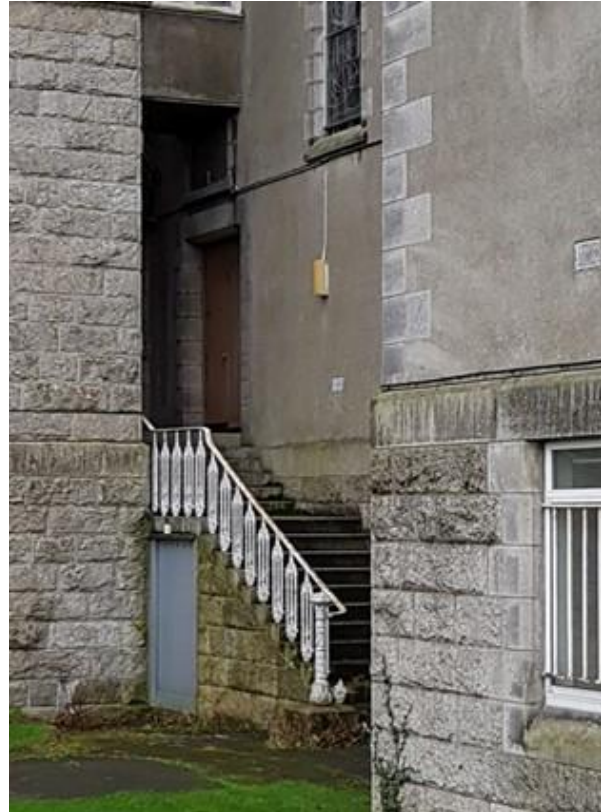
Plate 28: Cast iron balustrade on stairs to 1st floor
