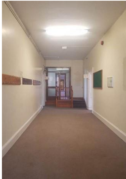
Plate 127: Corridor at same level viewing west to east
