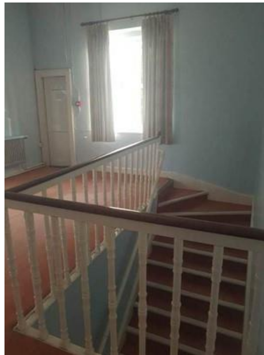
Plate 115: Stair access to lower levels
