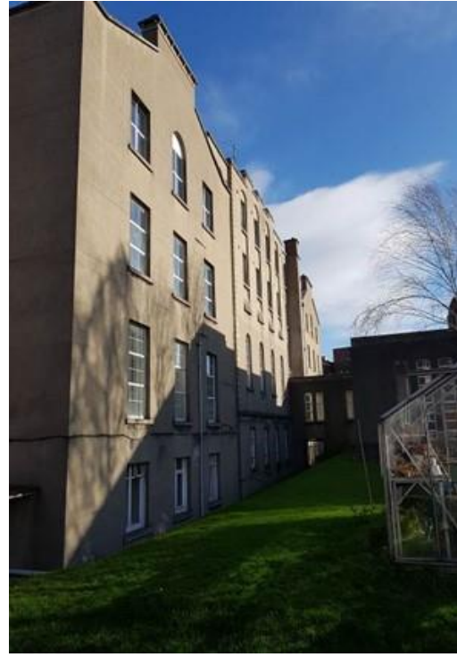
Plate 13: The rendered south elevation of the rear extension
