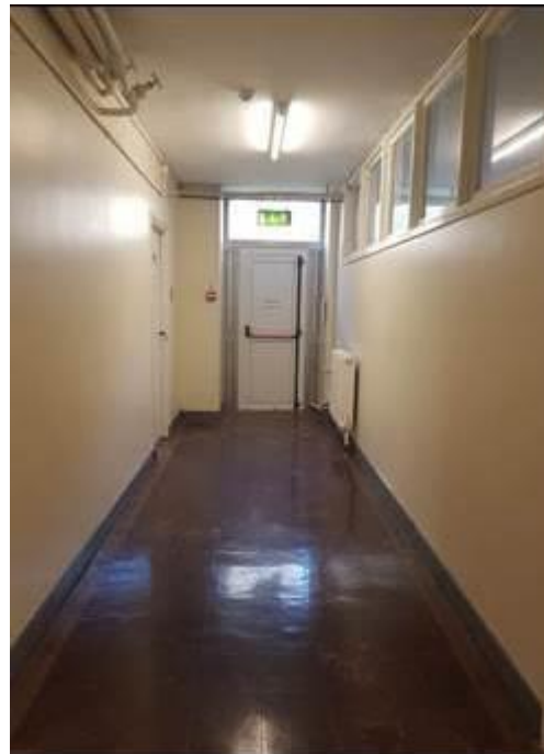
Plate 254: Corridor with fire door exit within the Finlay Wing
