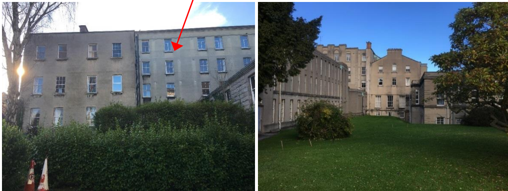
Fig.19 North elevation of Milltown Park, which was vertically extended in the late 19 th century. The north elevation of its rear, higher, extension was constructed in the 20 th century.
