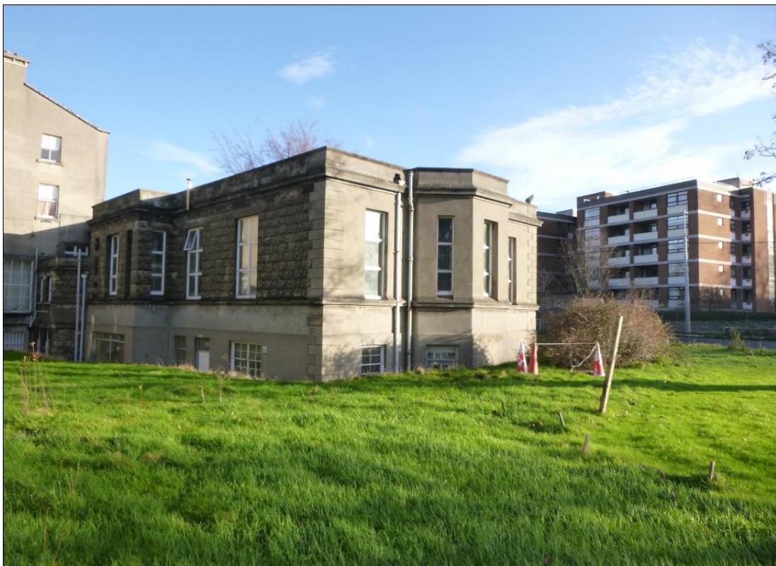
EASTERN SECTION OF SOUTHERN BOUNDARY – LOOKING NORTH EAST
