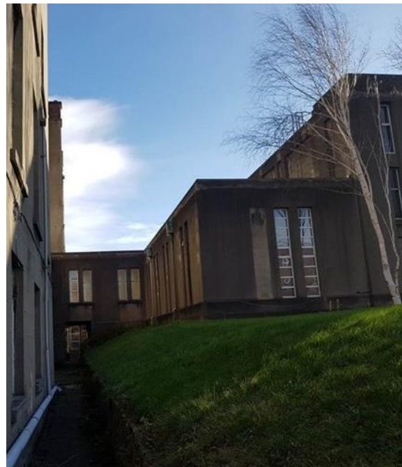
Plate 56: South west elevation showing the connection of the Archive wing to the Rear Extension. Note 1930's metal window frames
