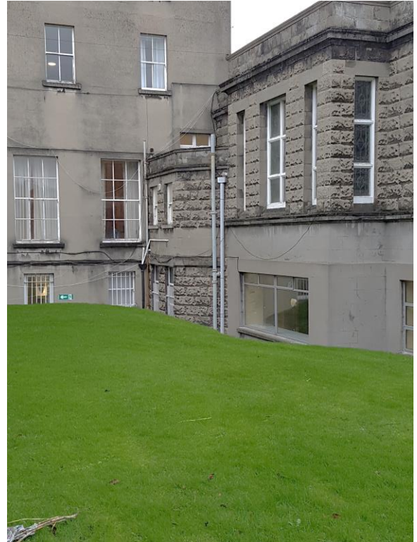
Plate 6: As above with view north east towards rear of Finlay Wing (1908)
