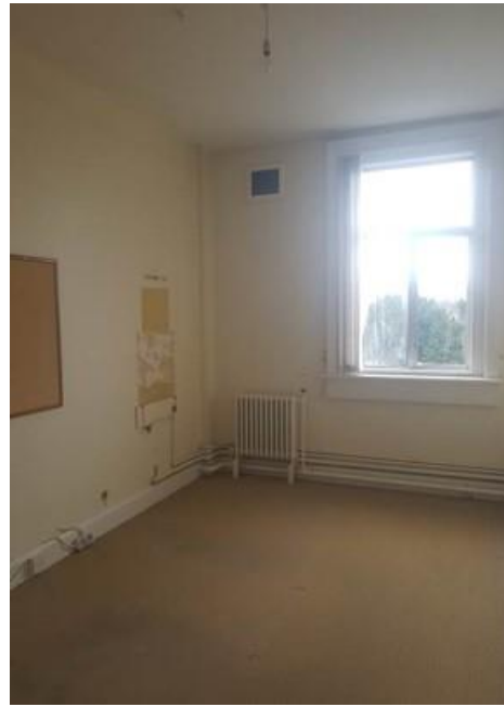
Plate 148: A typical dormitory
