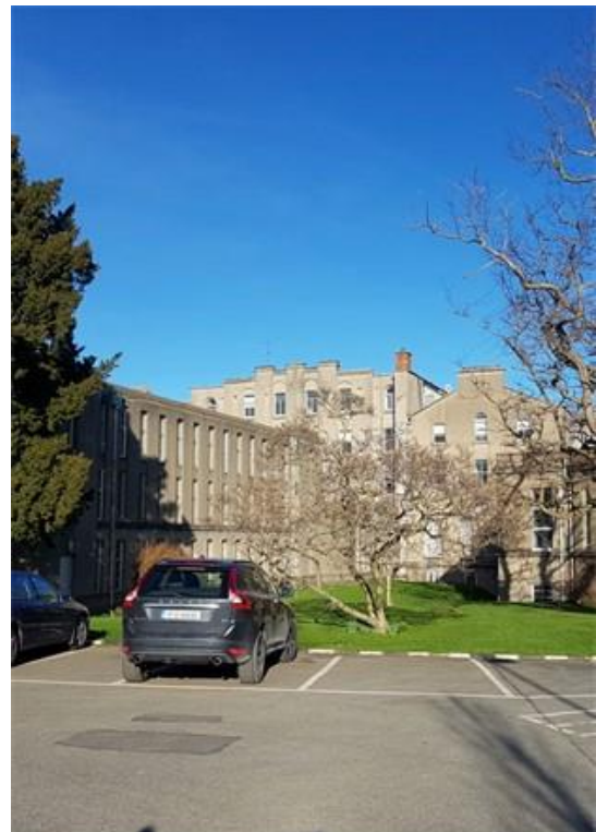
Plate 8: View of building range on entering Sandford Road gates from south
