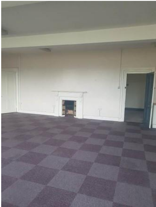
Plate 151: Large lecture room with fireplace at first floor level
