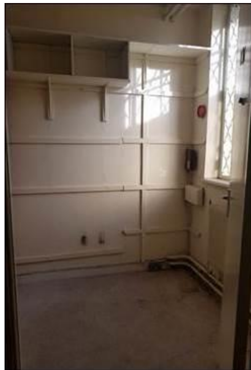
Plate 258: Large storage room
