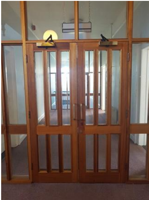
Plate 212: Opposing view from third floor
