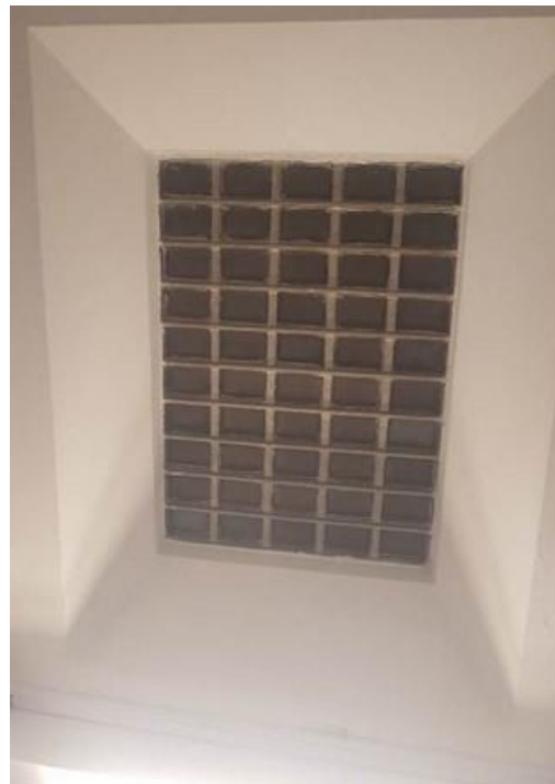
Plate 165: Example of cast iron rooflight at 2 nd floor level
