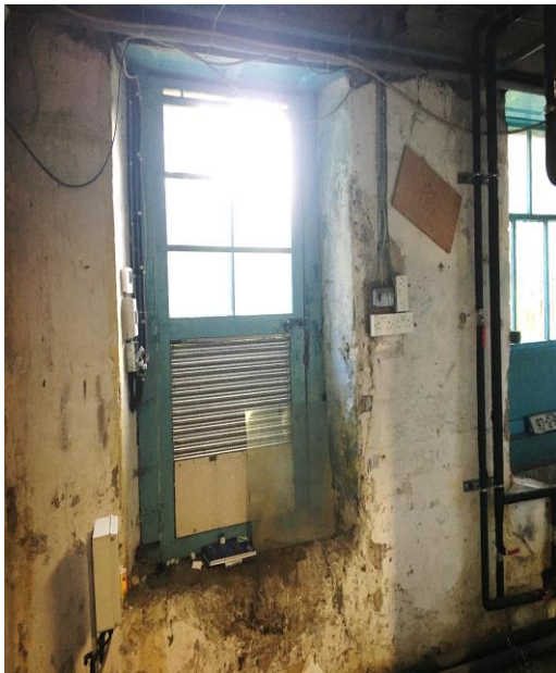
Plate 96: Original window at basement level
