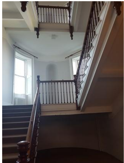
Plate 193: View up stairs at rear/north west side of building
