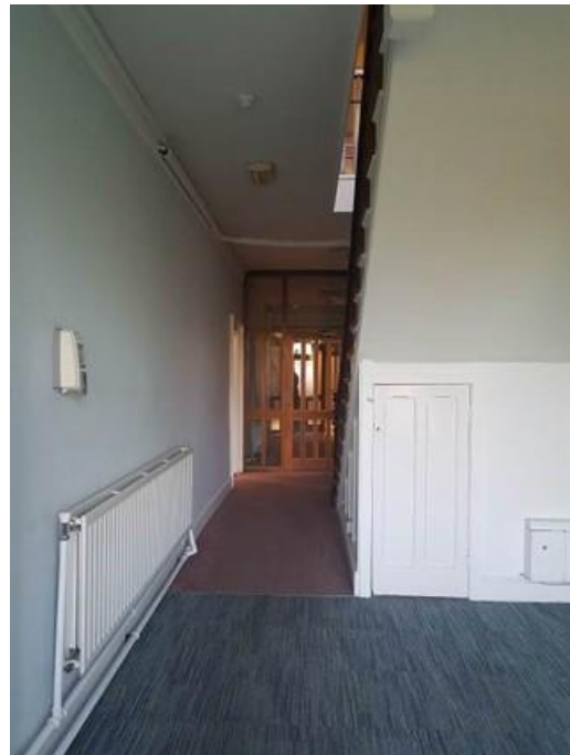
Plate 177: View from interior of side door, down corridor to main house
