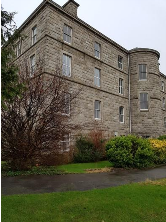
Plate 23 West elevation with bowed bay
