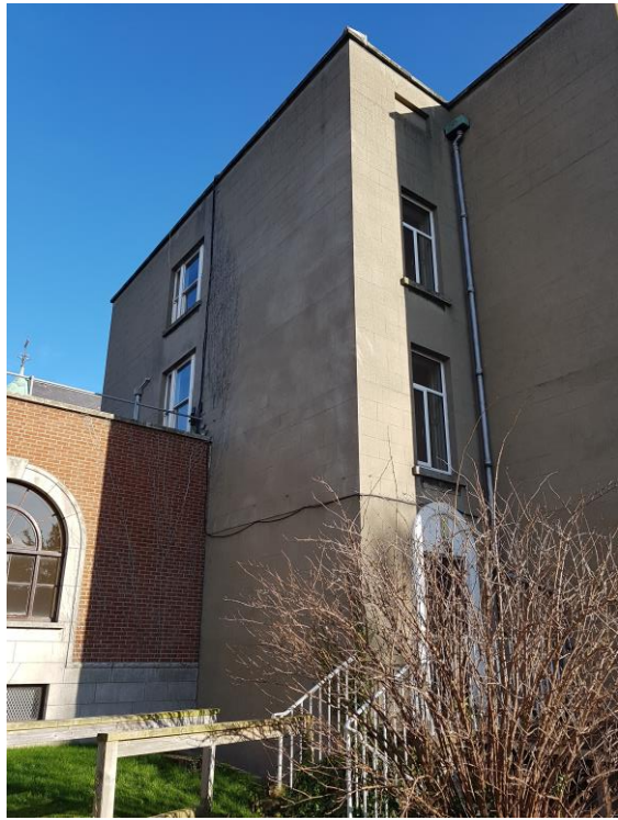
Plate 63: Rear extension connection to red brick, link building, viewed from SW.
