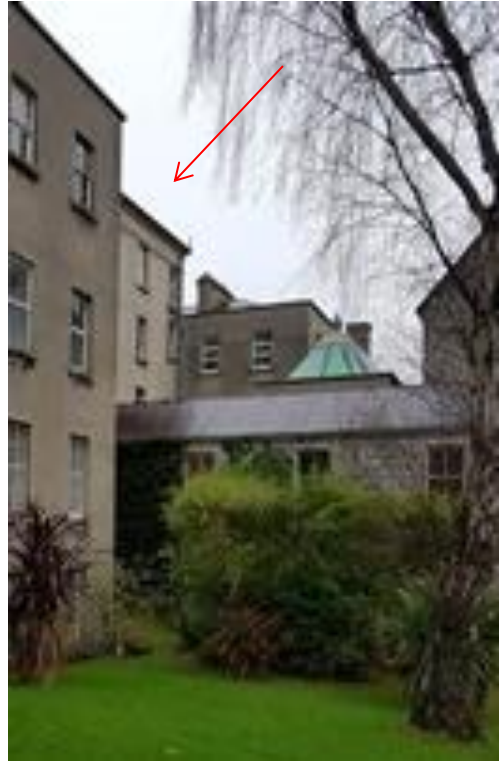
Plate 10: View west of the same elevation with the rear extension, link building and turret of small Sacred Heart Chapel (1911) in view
