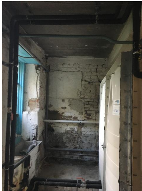
Plate 97: Original masonry walls within same plant room
