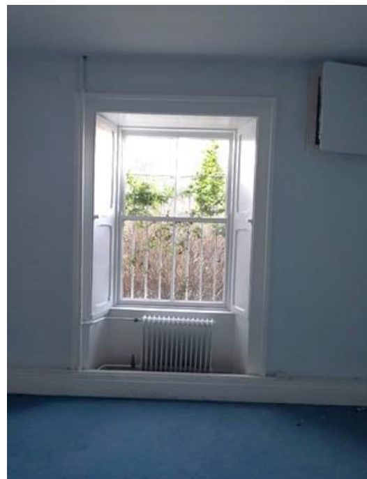
Plate 181: Lower ground floor bedroom
