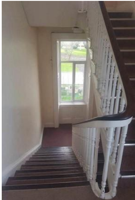
Plate 139: Stair linking 1 st and entrance level of rear extension block
