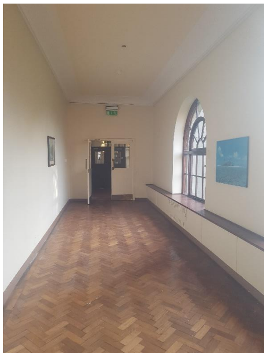
Plate 275: As above, opposing view towards entrance door
