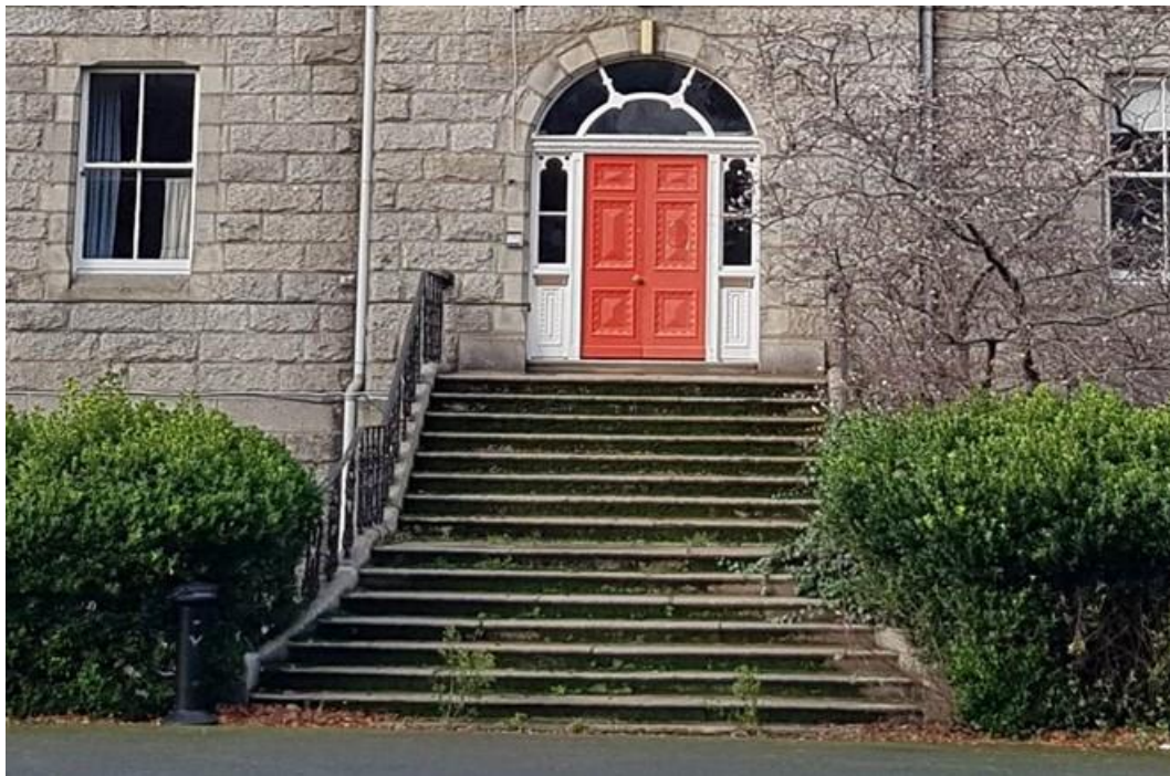
Plate 19: Original panelled front door and granite steps to Tabor House
