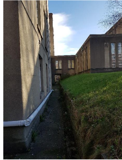
Fig.49 West elevation in context with Extension Block
