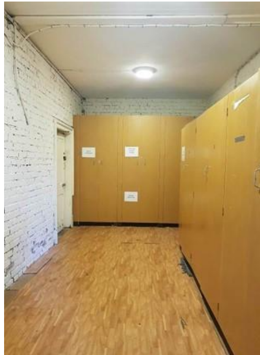
Plate 185: Services area at basement level
