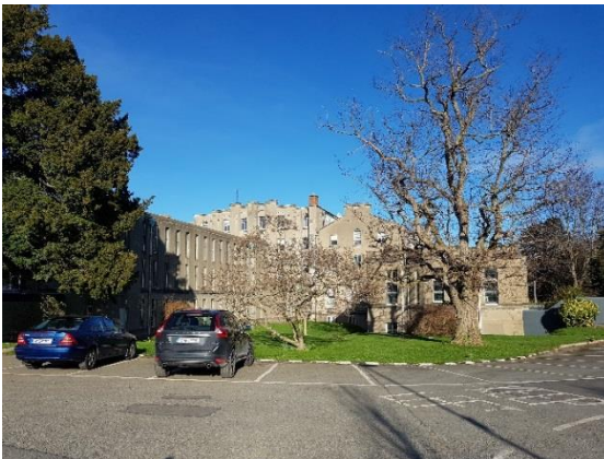
Fig.52 South elevation in context with the grouping
