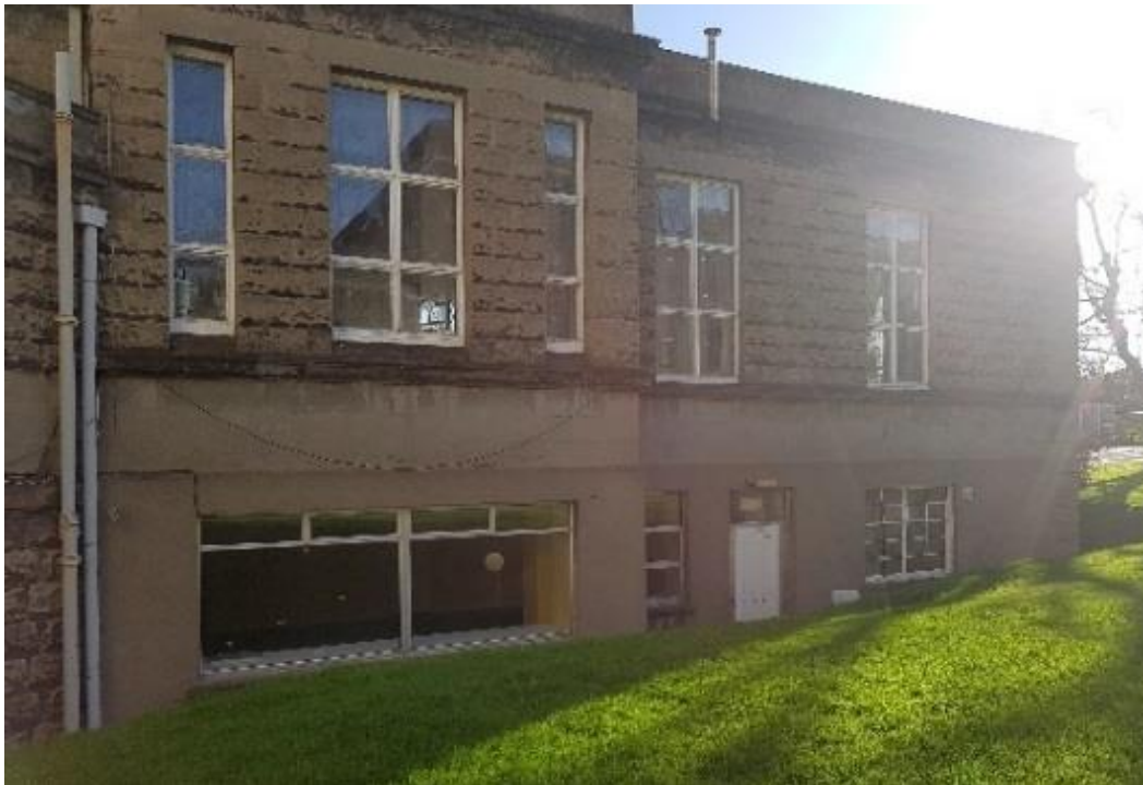
Plate 46: View of west elevation
