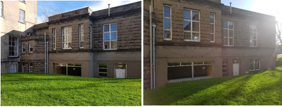
Fig.41 View of west elevation
