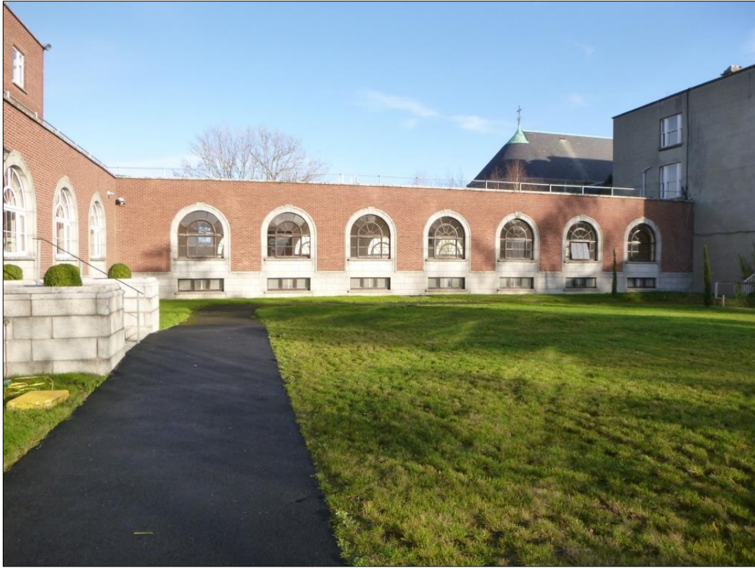
CENTRAL SECTION OF SOUTHERN BOUNDARY – LOOKING NORTH
