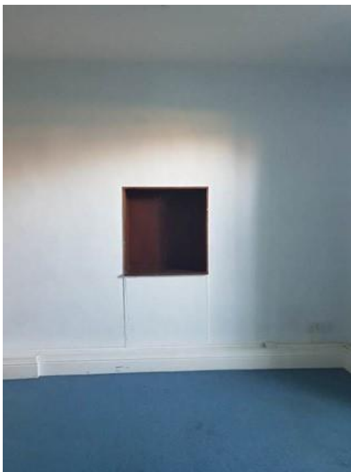
Plate 180: Access to dumb waiter now covered
