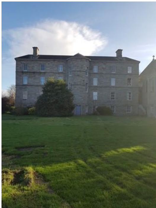
Plate 21: Tabor House west elevation in context
