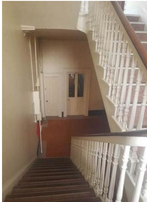
Plate 140: Stair linking 1 st and entrance level of rear extension block
