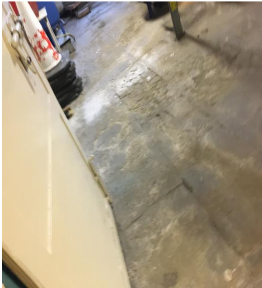
Plate 94: Flagstones in original kitchen at basement level
