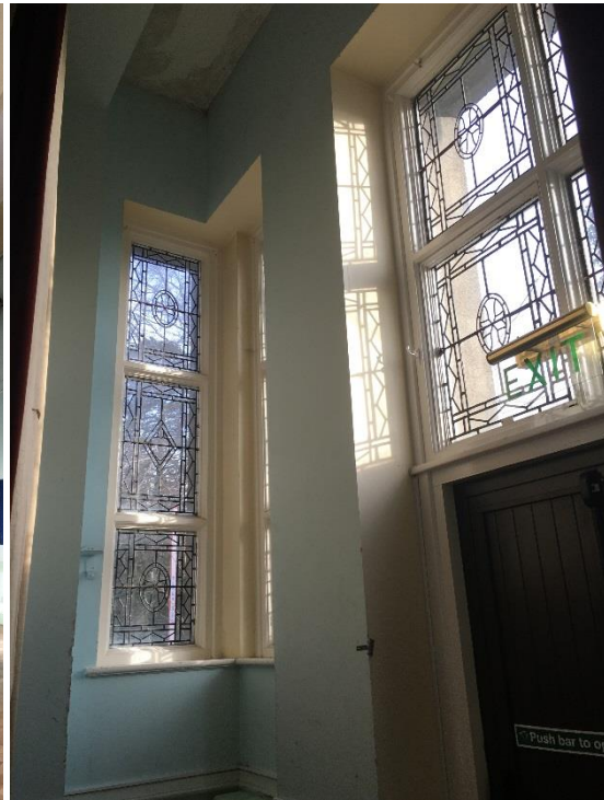
Fig.44 Leaded windows within lobby to east
