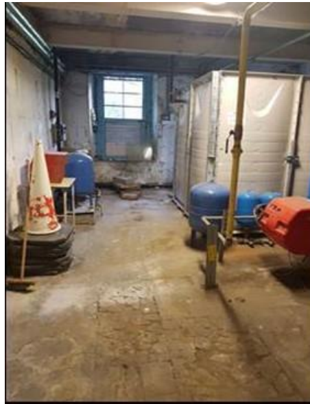
Plate 95: Basement level plant room, a former kitchen, under existing reception room
