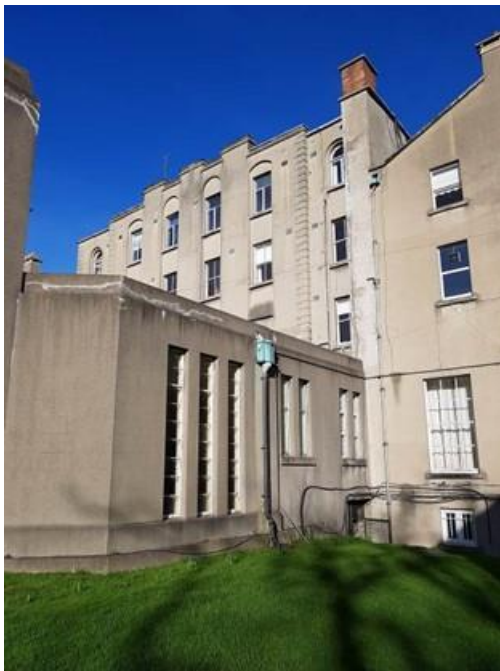
Plate 55: As above closer view of the Link to/from the Archive wing
